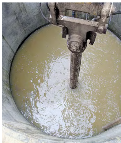
Tremie concreting to create a watertight seal
