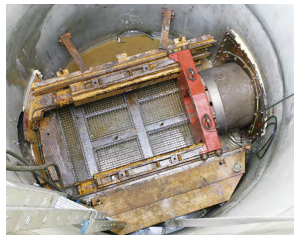
Pipe jacking system
